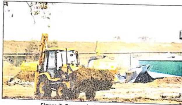
Figure 7: Removal of contaminated soil
