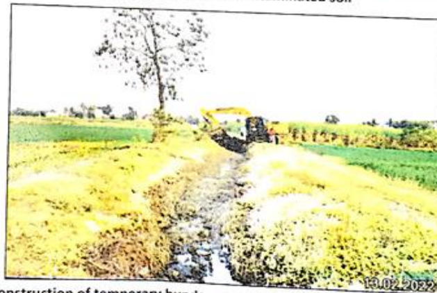
Figure 8: Construction of temporary bunds on natural drain to restrict the flow of molasses
